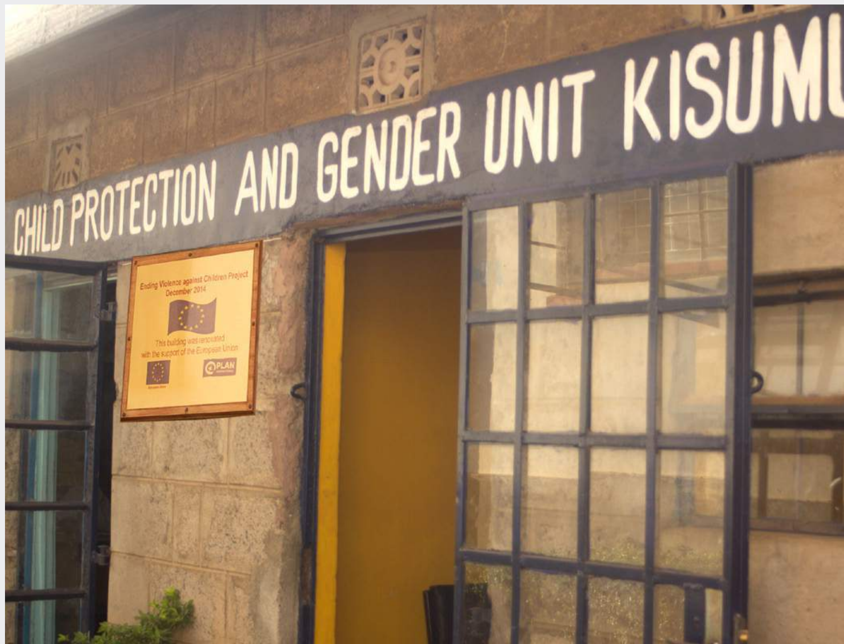
A building that houses the child protection and gender unit at Kisumu Central Police Station. It was renovated by Plan International under the EUVAC project
